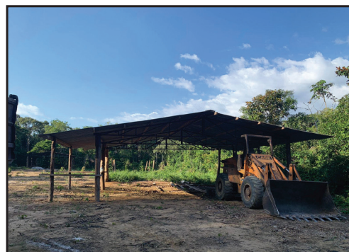
Camp structure being built
