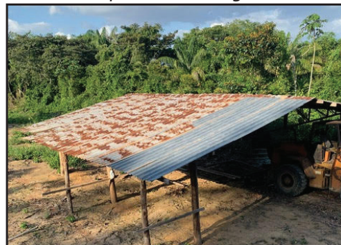
Camp structure being built
