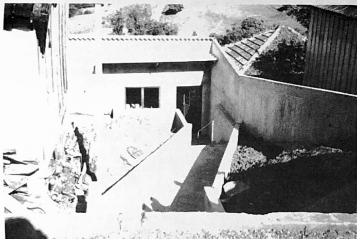
This is the new building at Santa Terezinha. In foreground you see the ramp and stairs that lead to the auditorium with seating capacity of 120 persons. Built on very declining land, this part was built with foundation that supports two more stories. In the future there can be built another floor for educational space and on top, an auditorium to seat 300 persons.
