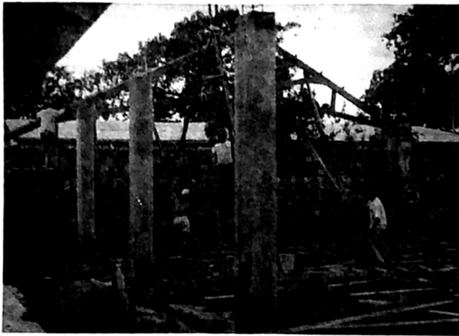
Pulling up the first roof truss for new First Baptist Church building. Iquitos, Peru. James Kissel with hat on at right.
