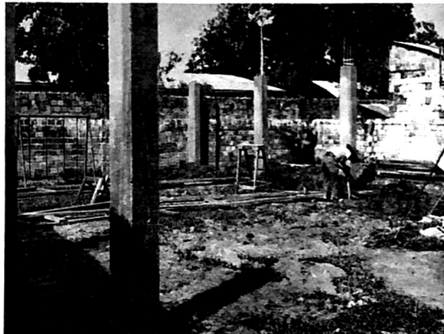
Concrete columns with four steel rods in each one for reinforcement for new First Baptist Church building, Iquitos, Peru, being built by James Kissel. See next page for more pictures.
