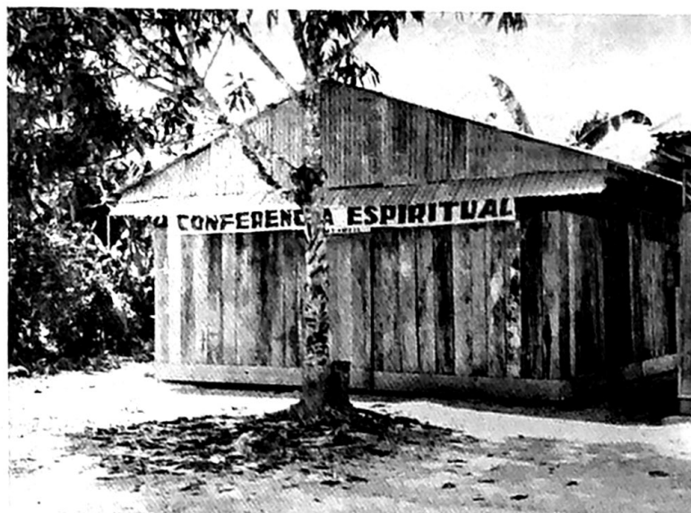
New building built by James Kissel and some of the men at Santo Tomas, interior near, Iquitos, Peru. Rough timber, metal roof and dirt floor.
