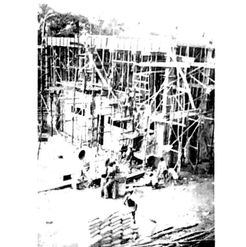
Pouring the concrete ceiling of the second story of Harold Bratcher Church building, Manaus, Amazonas, Brazil.
