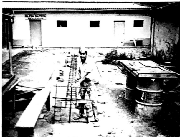
Brother Maglorio helping to tie the steel rods for the concrete columns of Art Gibbs's church building, Huanuco, Peru. Note the temporary church building in the rear. This building will have a concrete roof.
