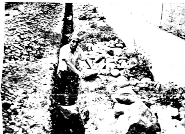
Brother Maglorio is digging the trenches for the concrete footings. He thinks he needs help for the big rock in the trench in front of him.
