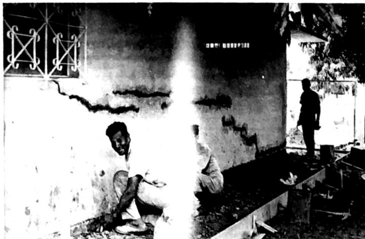
Cracks in one side of Mayfield house, Pucallpa, Peru being repaired, and forms for sidewalk.
