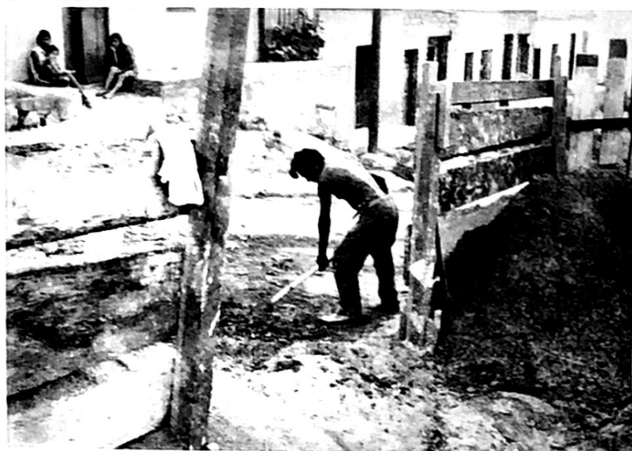
LAUERMAN CHURCH BUILDING IN TEGUCIPALPA. Making concrete mixture for the concrete rock wall.
