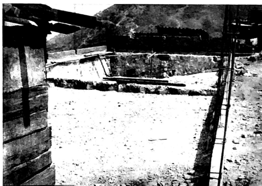
Honduras building project. Note the partly finished concrete wall in the rear. Note steel webbing for reinforcing concrete pillars.
