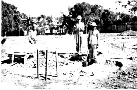
Digging the trenches for the footings for the new church building in Pucallpa, Peru. By the time you read this the foundation will perhaps be in and the wall partially up. Brother Mayfield hopes to complete as soon as possible.
