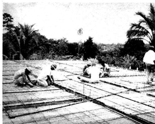
Wiring the steel rods for reinforcing the concrete second floor of the preacher's School Building in Manaus, Amazonas, Brazil.
